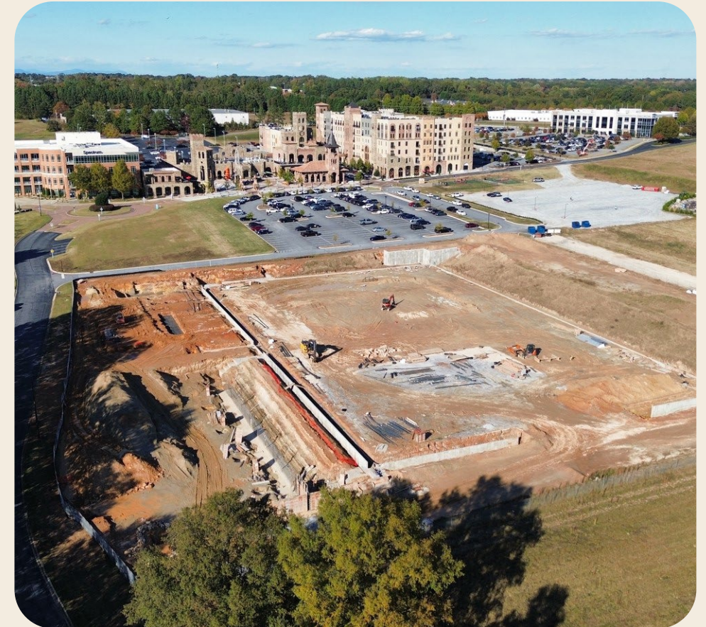
Stadium under construction at BridgeWay — October 2025.
